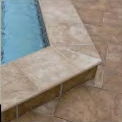
Raised pool beam and double sided coping.
